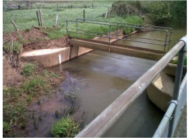
Water abstraction point at Burnt House pumping station
